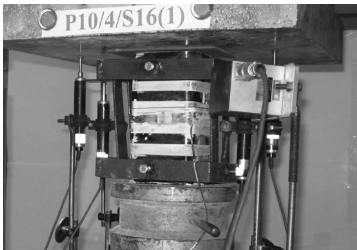
Figure 2- Setup of axially test of a prismatic specimen
