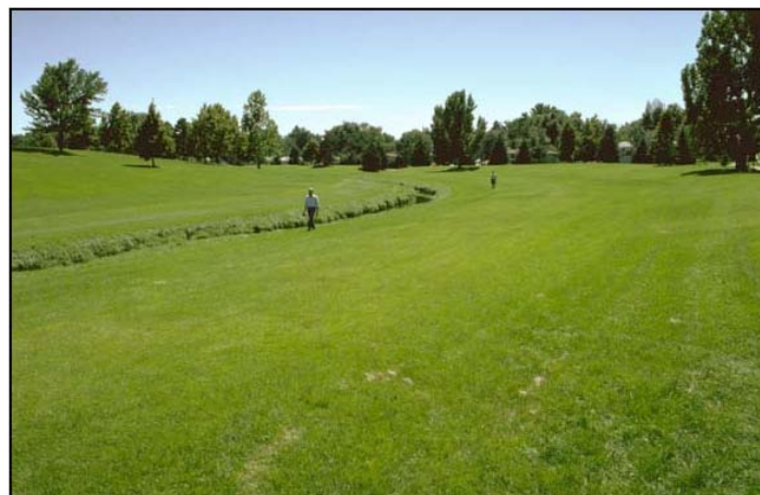
Figure 2- A wide-open waterway carries floodwater at modest depths while maintaining low velocities to inhibit erosion.
