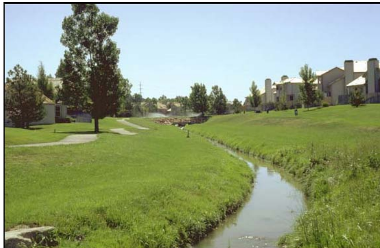
Figure 1- Use of uniform design standards represents a reasonable standard of care for urban flood channels.
