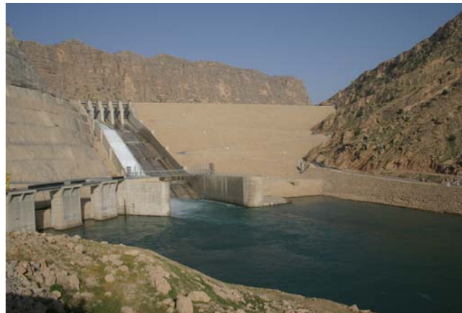
Fig1. Masjed Soleyman embankment dam view
