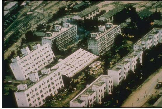
Fig.7. Tilted buildings; bearing capacity failures, 1964, Niigata- Japan
