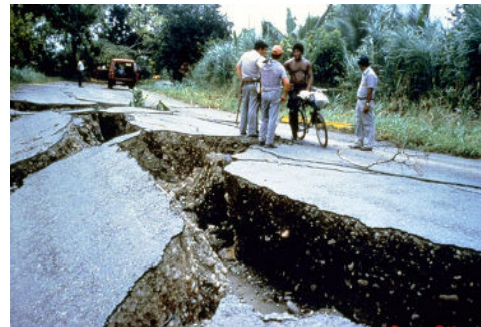
Left - Fig.4. Earthquake Liquefaction damage, January 1996, Kobe-Japan
