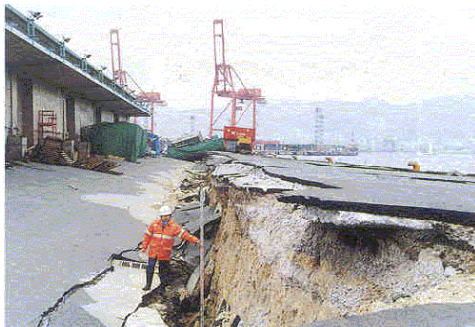
Left - Fig.4. Earthquake Liquefaction damage, January 1996, Kobe-Japan
